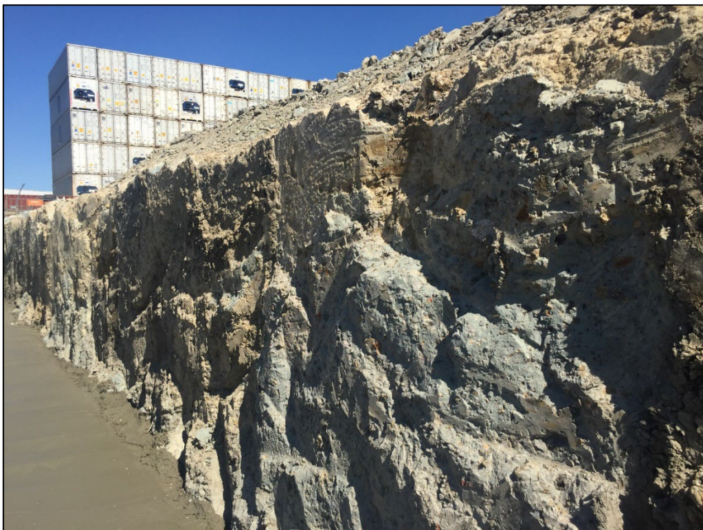
Fig. 5. Excavated face of CSM block
