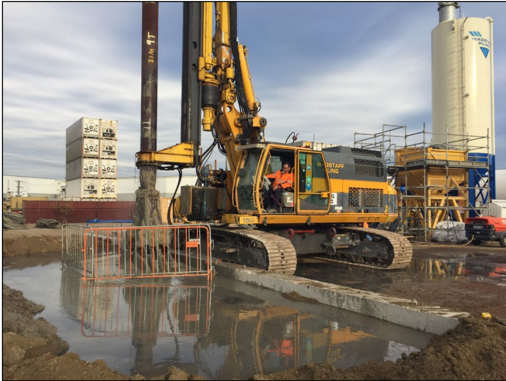
Fig. 4. Installation of CSM panels
