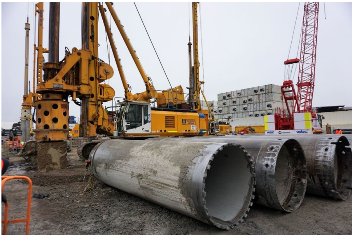
Fig. 9. Double wall segmental casing
